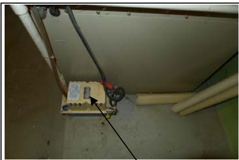
Condensate Pump in Use
