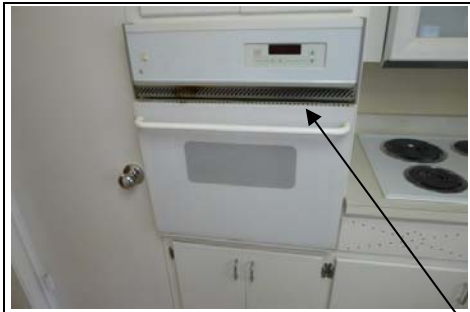
Electric Oven Door Damaged (sprung)
