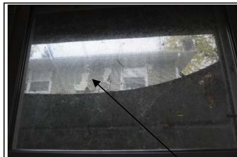
Repair Damaged Screen(s)
