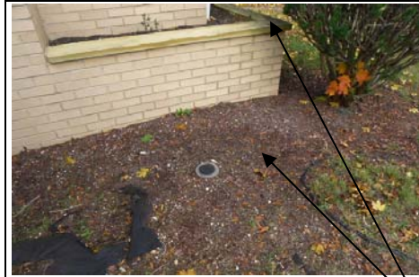
Tuck-Point Flower Box Mortar Joints Replace Wood Chips w/Stones
